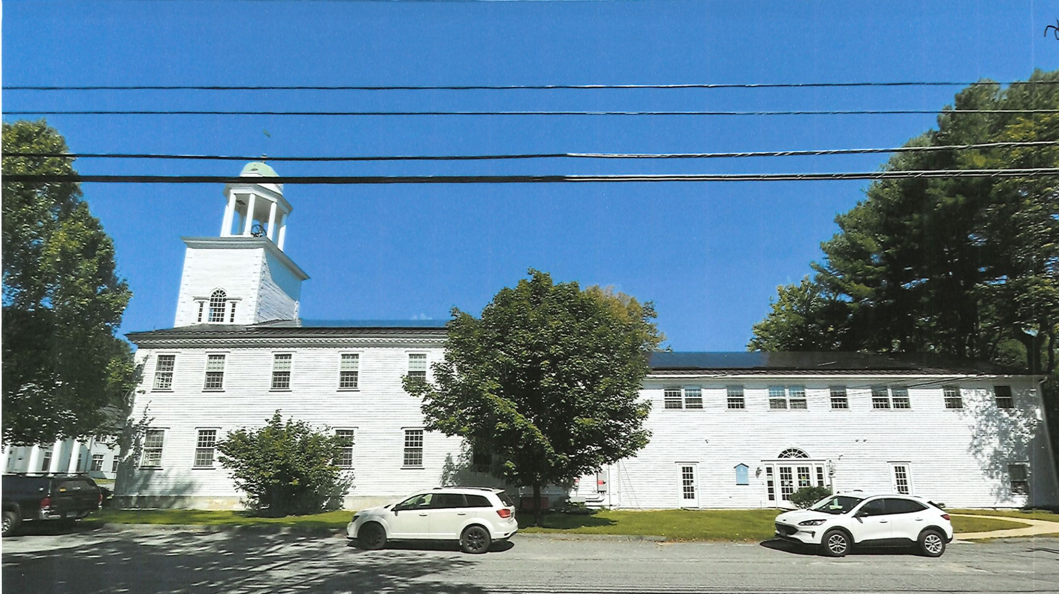
Salisbury Congregational Church In a Historic District also Please note the low profile of the panels. Roof is a metal roof here.
