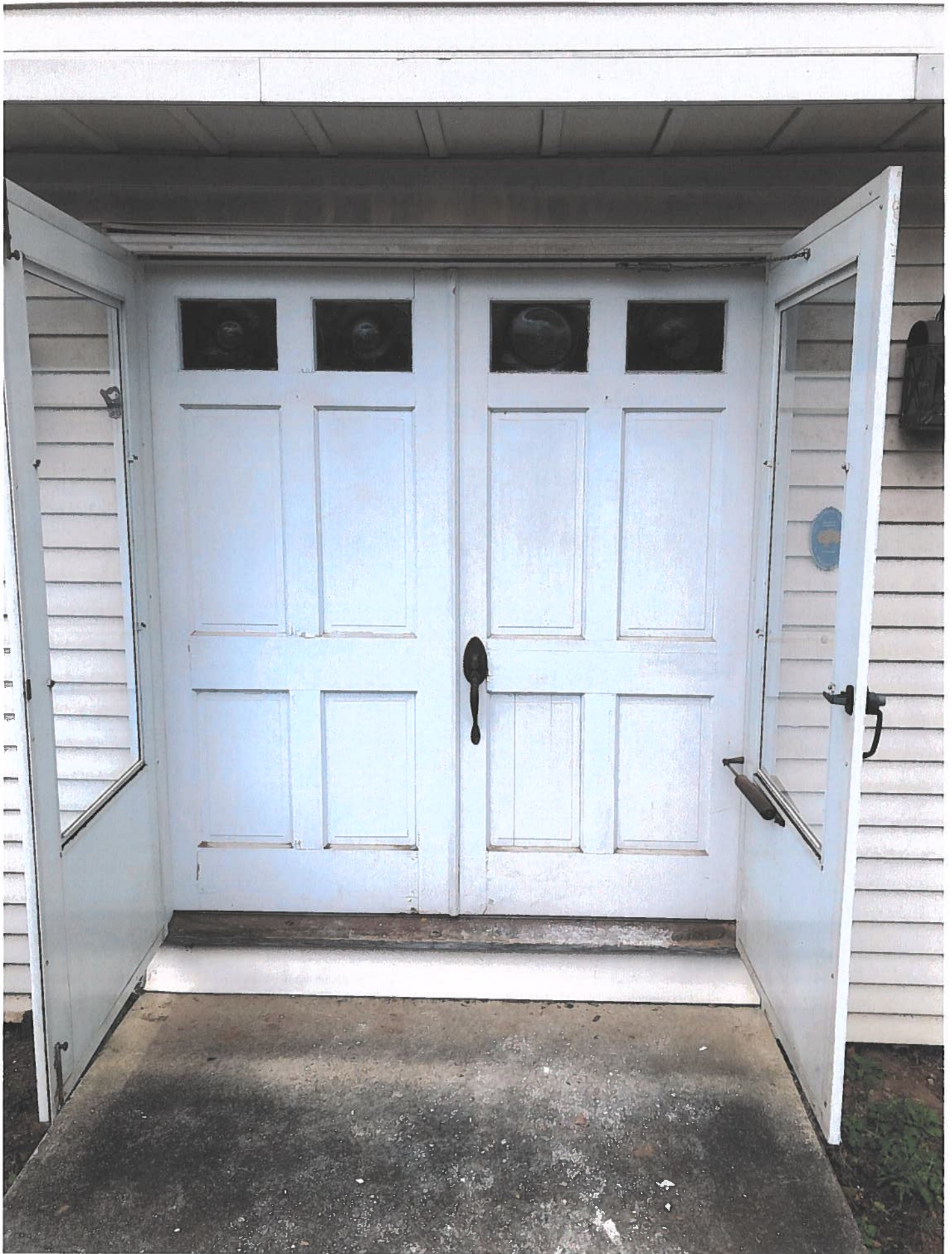
Existing Front Door
