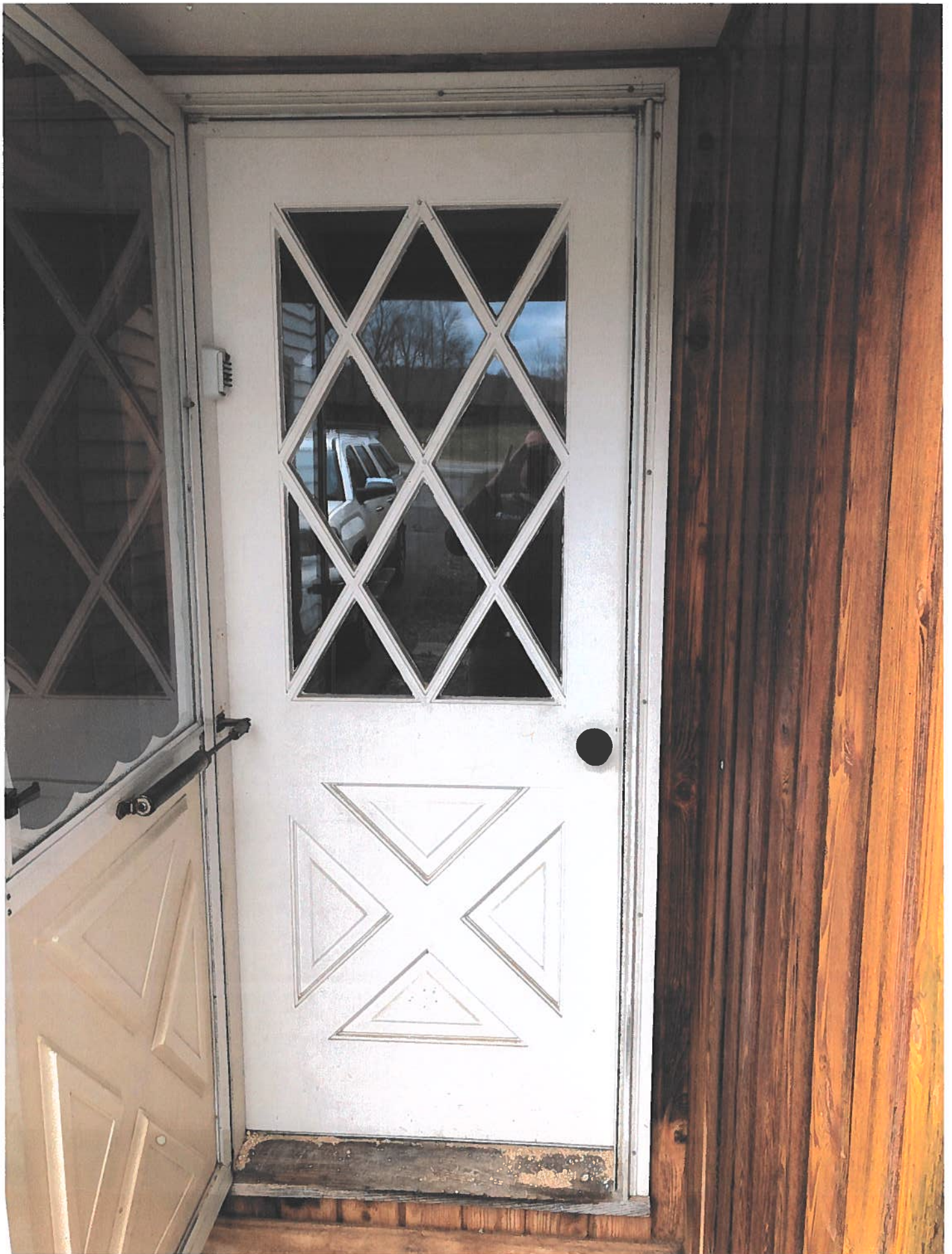
Existing Front Side Entry Door
